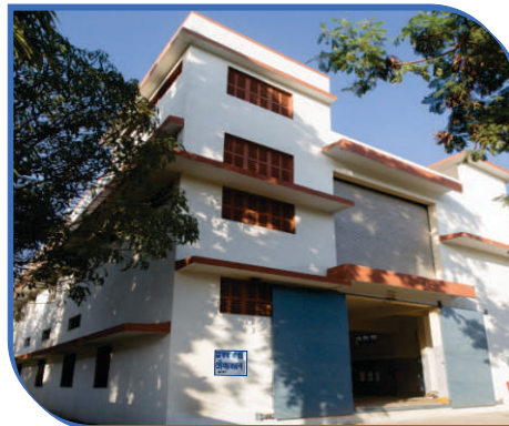
Office & Works Unit -IV
