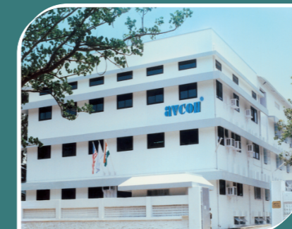
Office & Works Unit -II
