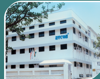
Office & Works Unit -II
