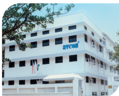
Office & Works Unit -II
