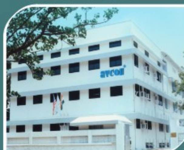
Office & Works Unit -II
