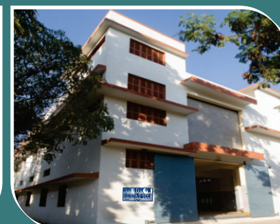
Office & Works Unit -IV
